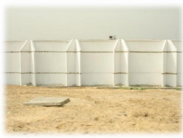
Final Stage of Fencing
