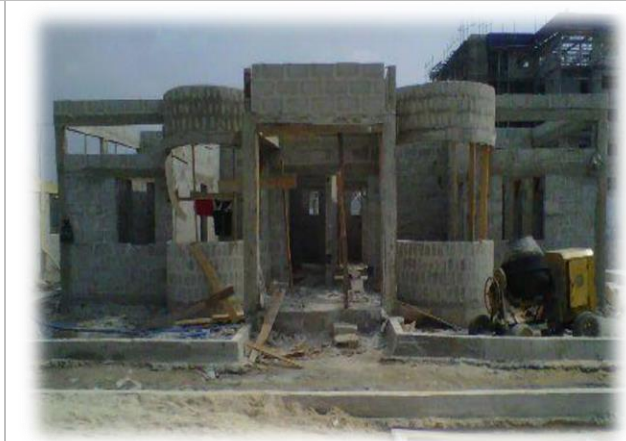
Lintel level of Delta Bridge Garden Park Eatery
