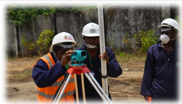
Survey team checking for the ground level.
