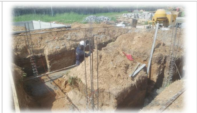
Blinding and Column Setting
