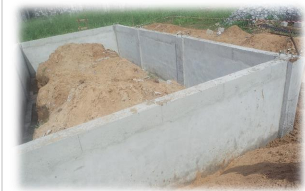
Casted Column Base Ready to be Sand Filled
