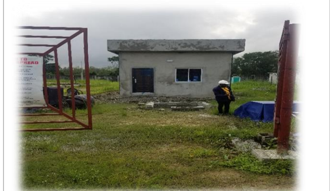
Completed Gate House
