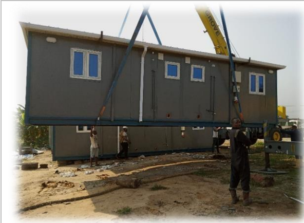
Lifting of Container (caravan) into the Flatbed
