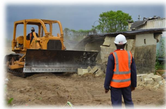
Clearing of Existing structures and Materials from Proposed Site for Construction
