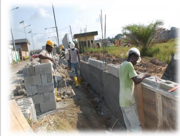
Form works on Fence
