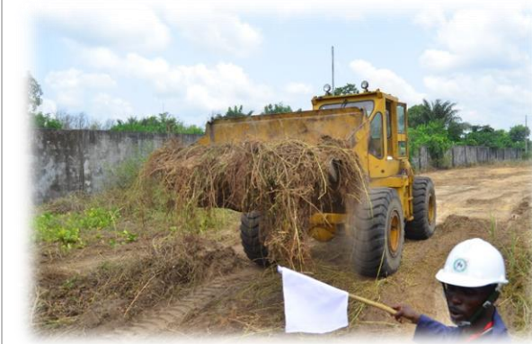
Land Clearing and preparation of Site
