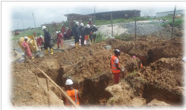
Setting Out and Excavation trench for Gate House
